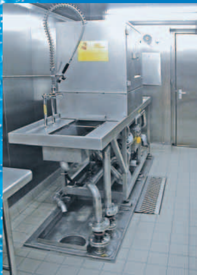
Built-in bone shredder in the food preparation area
