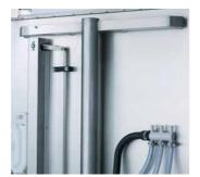
Pipework outwith the washing chamber (stainless steel).
